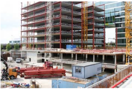
Figure 24 : Image showing the next building in the BARCODE being constructed.
