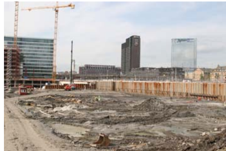
Figure 25: Excavated BARCODE site
