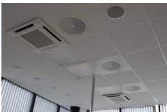
Figure 5: Conference room ceiling
